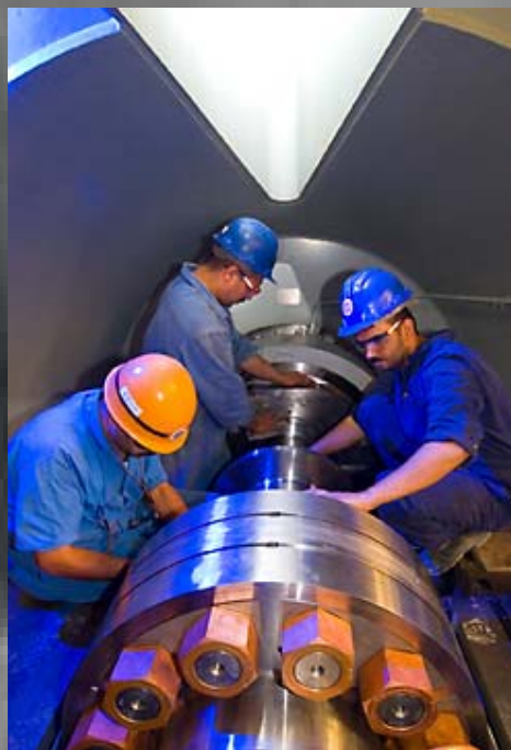
Steam Turbine Installation
